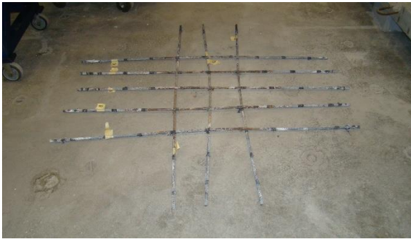
Figure 12: Corroded bars after demolition process
