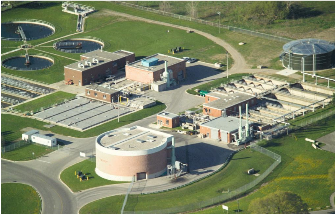
Figure 2.4. Adelaide wastewater treatment plant, London, ON, Canada
