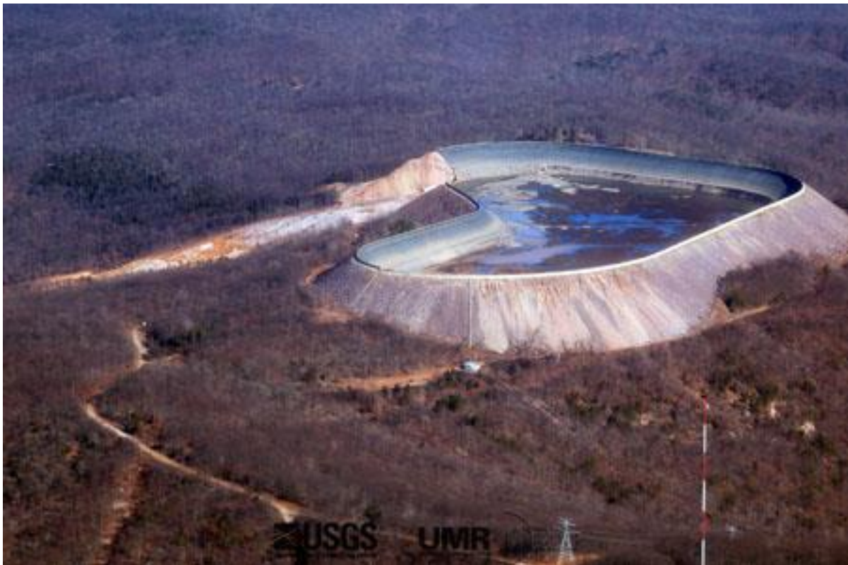
Figure 4. Taum Sauk Dam and upper reservoir after the wall breach, Lesterville, Missouri, US. ( https://commons.wikimedia.org/wiki/Category:Taum_Sauk_Reservoir_breach#/media/File:Taum_Sauk_upper_aerial-USGS-Picture037.jpg , last accessed on July 19, 2016)
