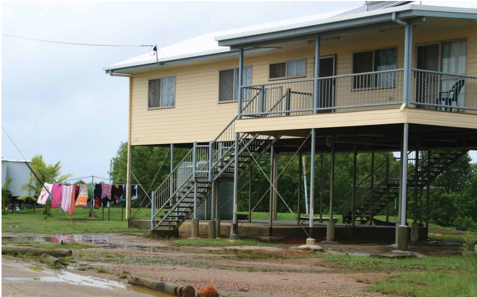
Figure 4. New raised house on Saibai.
