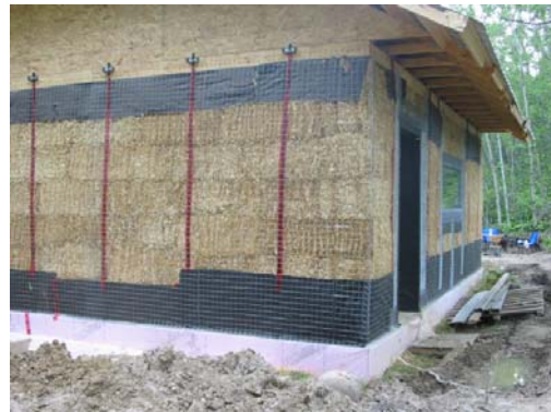
Figure 5-1: Straw Bale House in Construction
