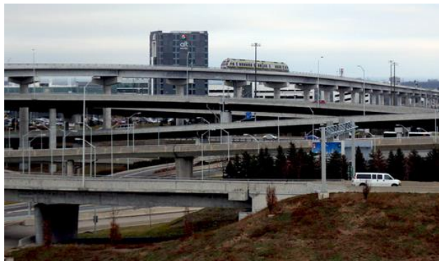
Figure 4: Existing bridges and Guideway
