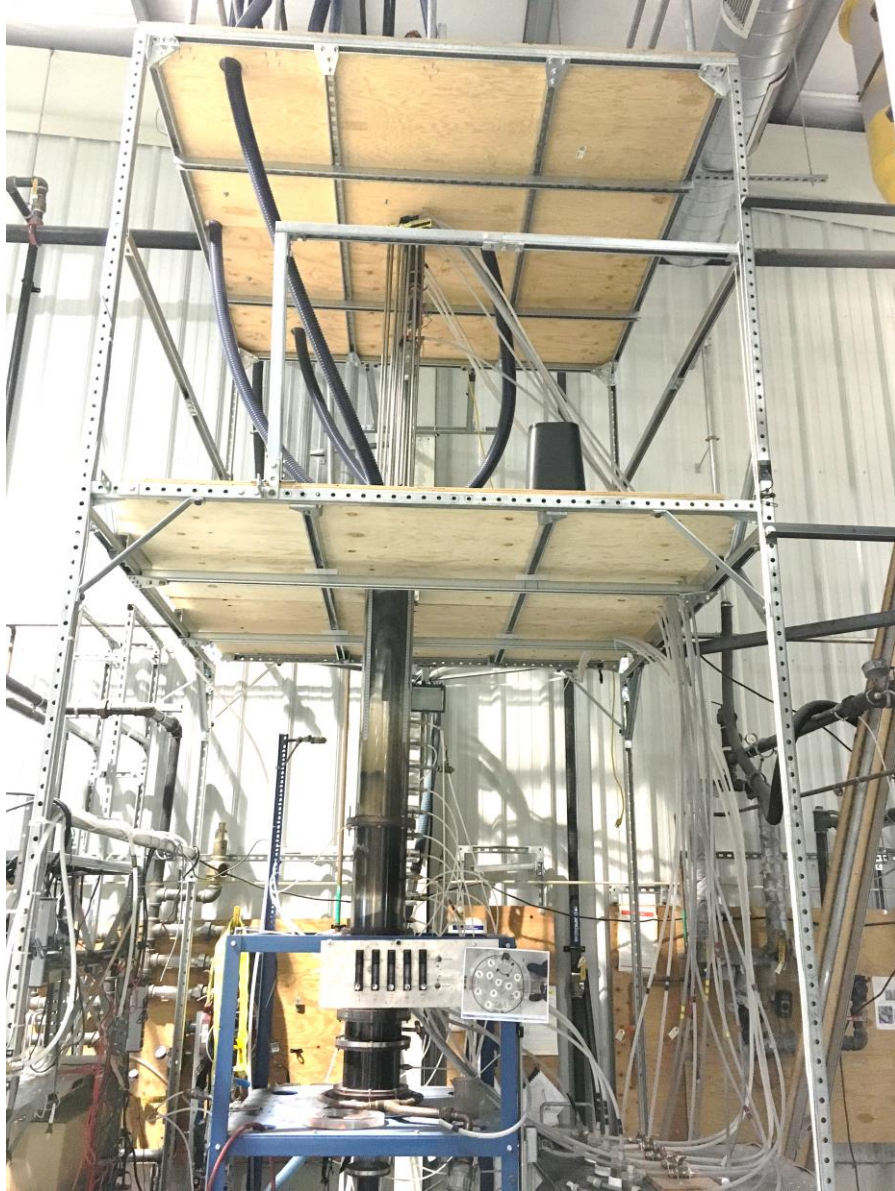
Figure 2-7. Internal and external supporting structures. Internal has a blue color, and the external is made of Unistrut®
