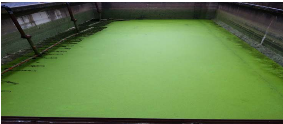
Figure 2.3: Eutrophication in a Decommissioned Aeration Tank, Taken Summer 2013 at the Adelaide Pollution Control Centre in London, Ontario, Canada
