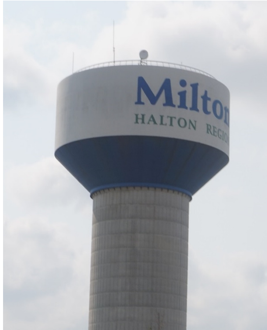
Fig. 3-1 Combined steel conical tank
