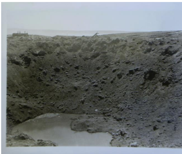
Photo 18 Picture showing one of the two major craters caused by the Bedford Magazine Explosion. This crater was made by ordnance improperly stored outside of the ammunition bunkers. LAC, RG24, Vol. 8070, File: 1270-41 Ammunition Disposal Committee, Bedford Basin, Colonel Ogilvie's Reports, Copy Negative HS 1509-64
