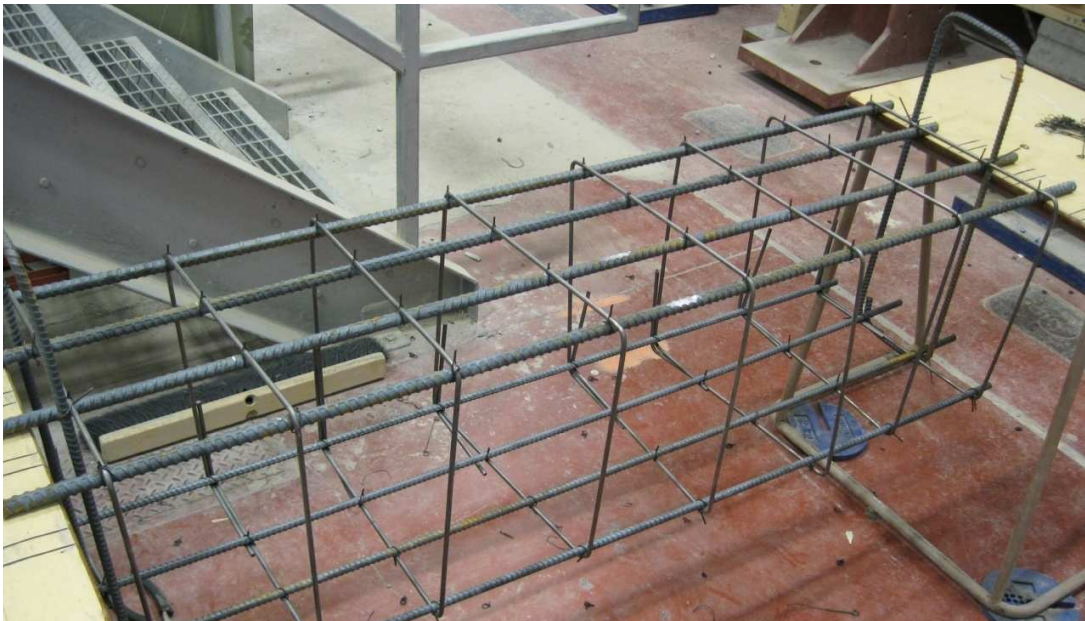
Figure B- 4 Rebar cage tying procedure
