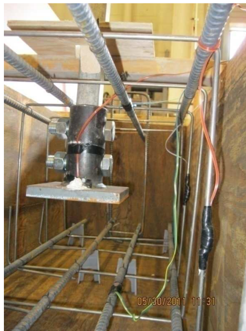
Figure B- 7 A ready system for concrete casting
