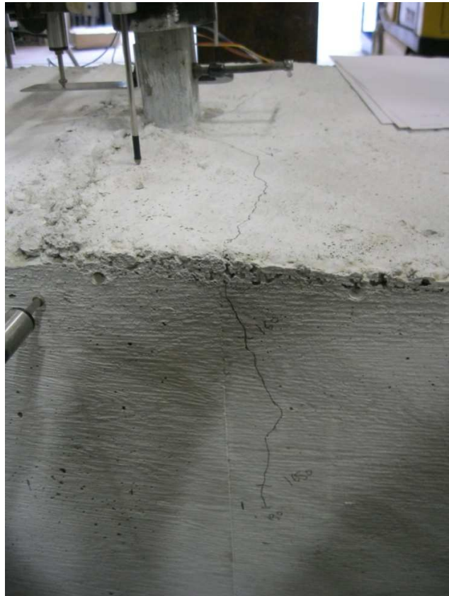
Figure 3- 6 First flexural crack initiation and propagation
