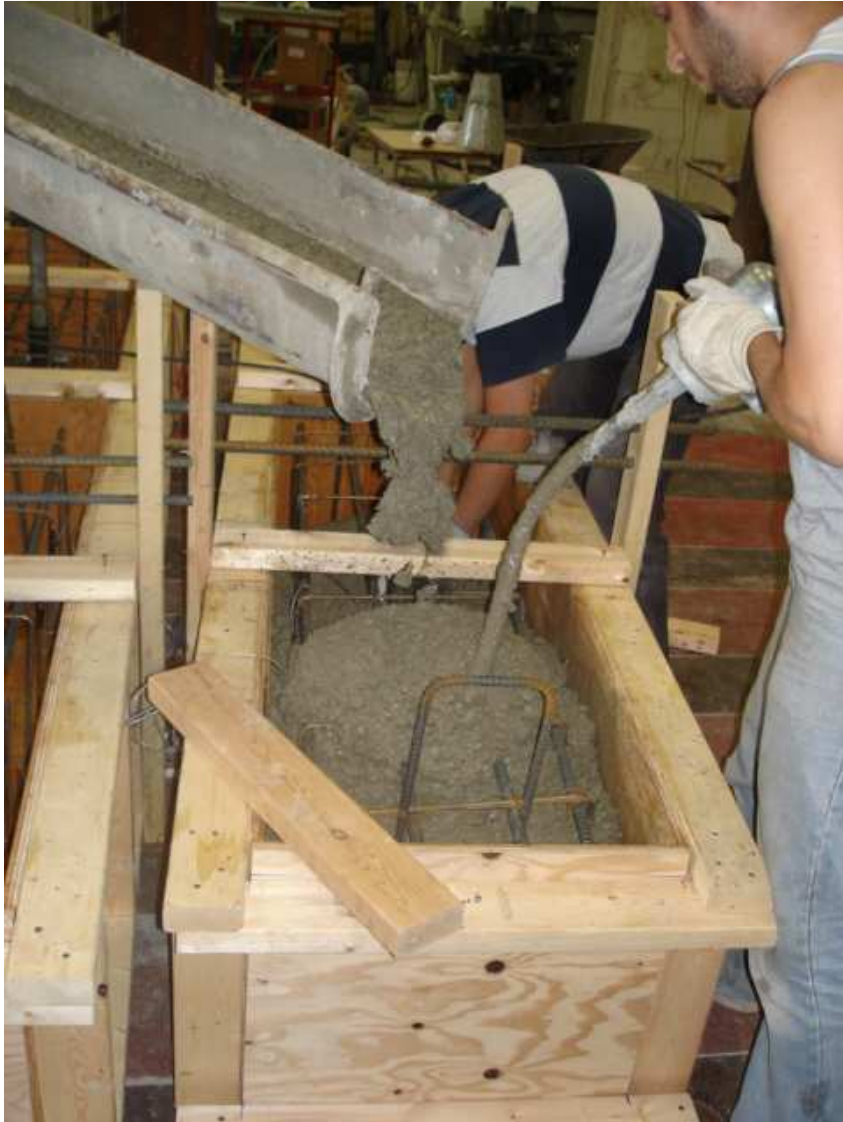
Figure B- 8 Ready mix concrete casting and concrete vibration
