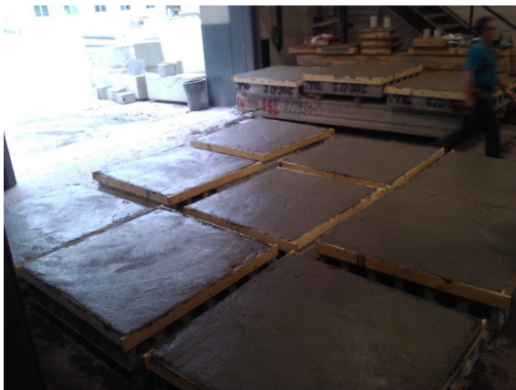
(c) After casting the topping (1 st shipment)
