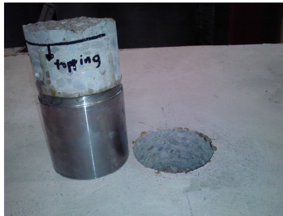
(c) Hollowcore slab failure (H)
