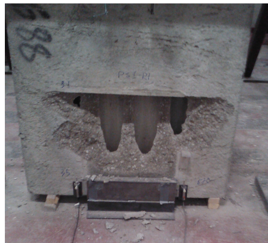
(b) Peel failure in hollowcore slab
