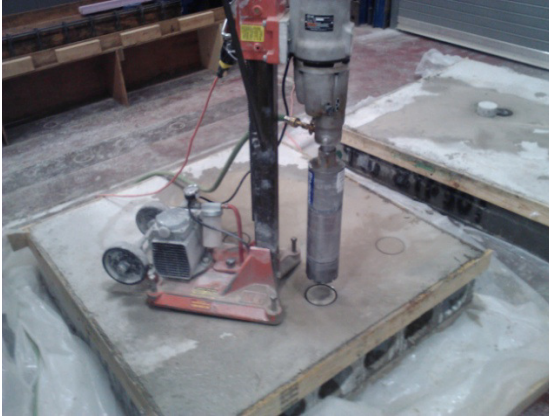
(a) Core drilling
