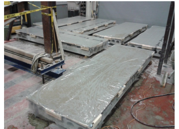
(f) Curing of the concrete topping
