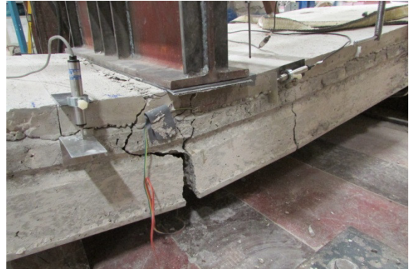
(b) FMA2-2C (strand rupture).
