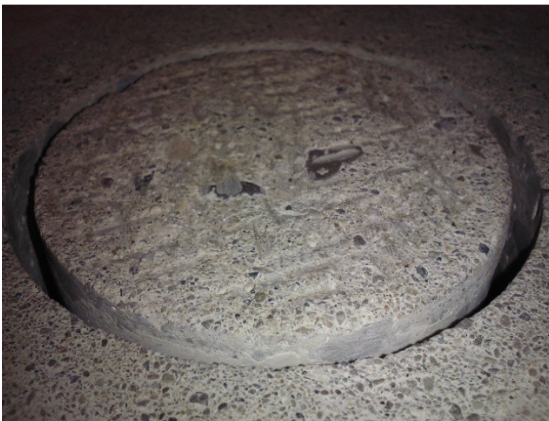
(c) Roughening of core surface
