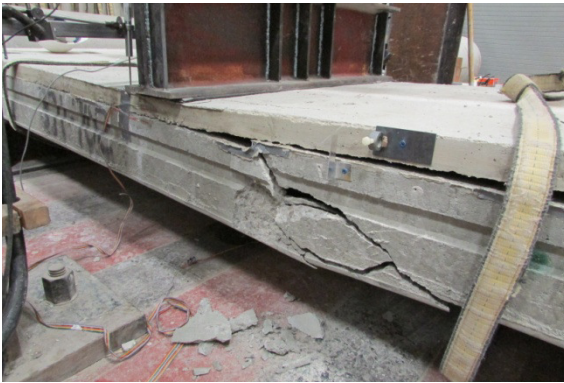
(c) FMB2-2 (flexure-shear failure).
