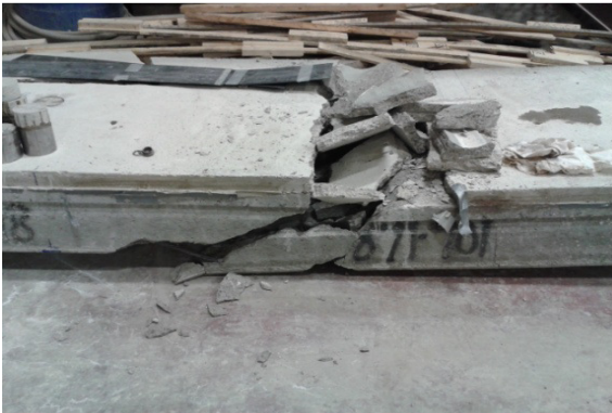
(e) FMB2-3 (flexure-shear failure).
