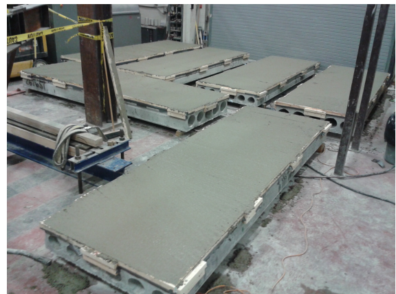
(d) After casting the topping (2 nd shipment)
