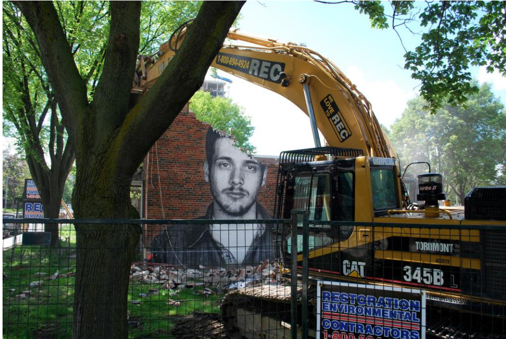
Figure 1.10: Image of Tyrone being destroyed by a backhoe as part of the Regent Park Revitalization Project (Regent Park, Toronto, Ontario, 2008). Photograph and permission courtesy Dan Bergeron / Fauxreel Studios.
