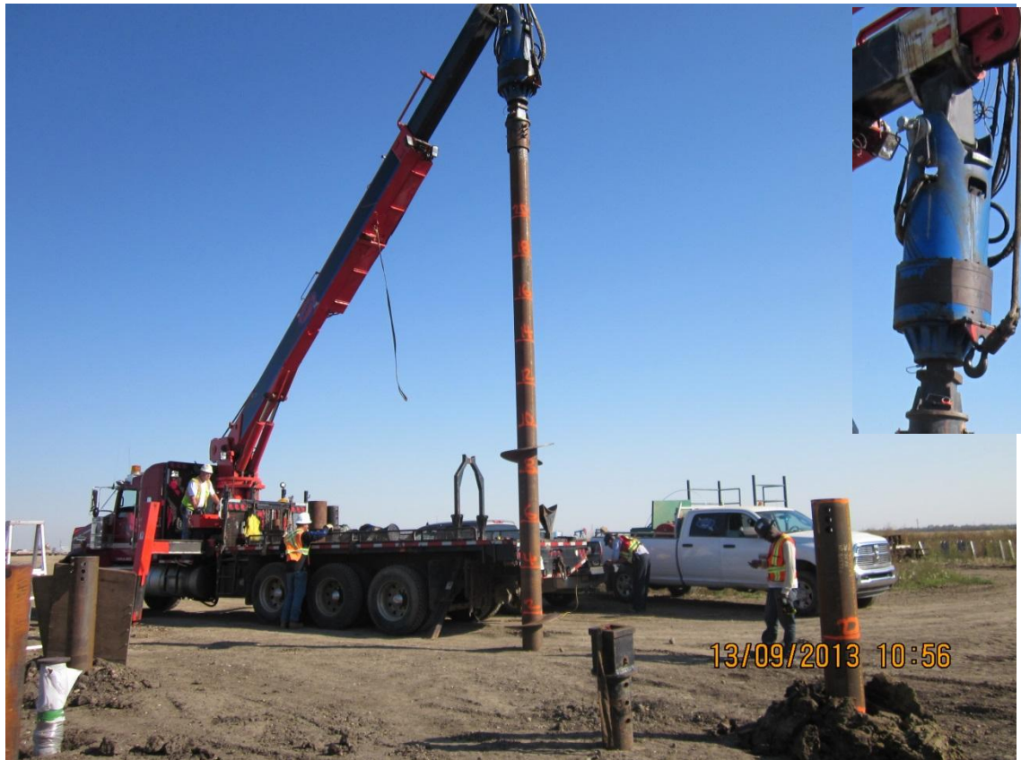
Figure 4-1: Boom Truck & Digger 1400
