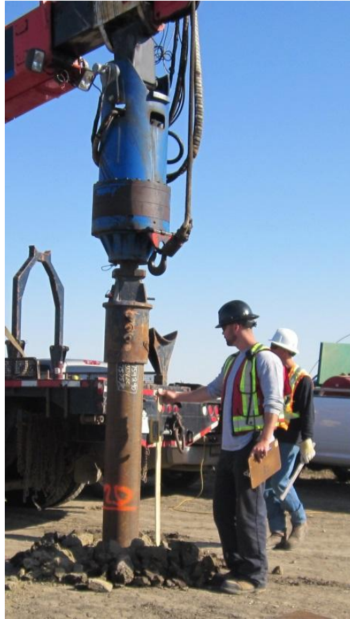
Figure 2-4: Digger 1400 & Boom Truck
