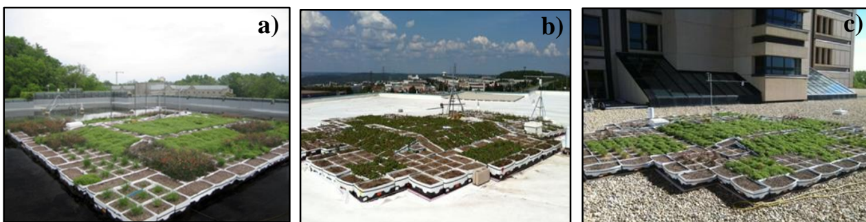
Figure 3. 1: Experimental green roofs in a) London Ontario b) Halifax Nova Scotia and c) Calgary Alberta
