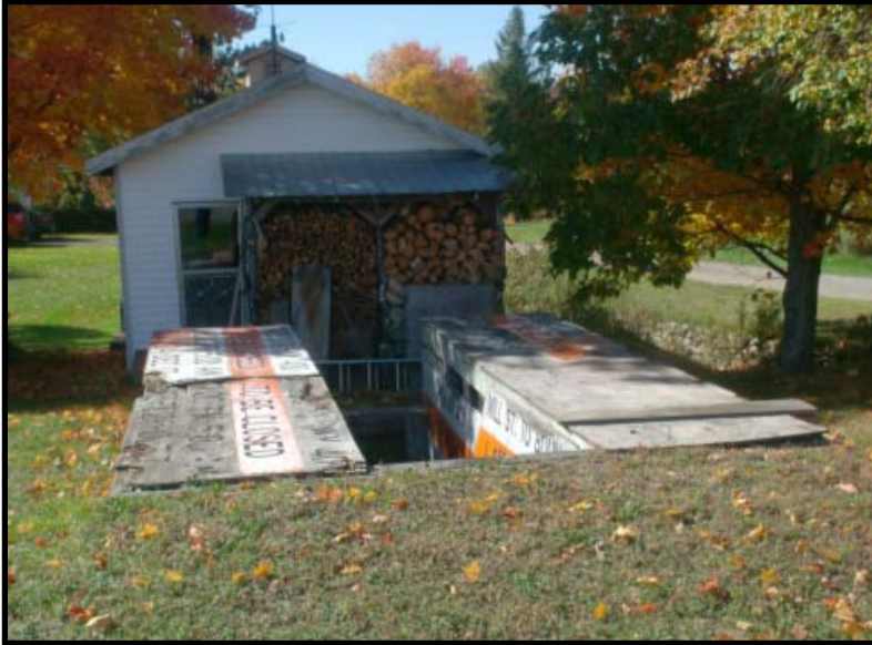
Figure 37: Oil Change Station Made from Reclaimed Highway Signs
