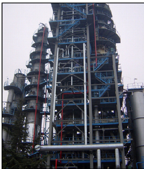
Figure 2–12: Industrial demonstration of a downer reactor (Jinan Refinery, SINOPEC).
