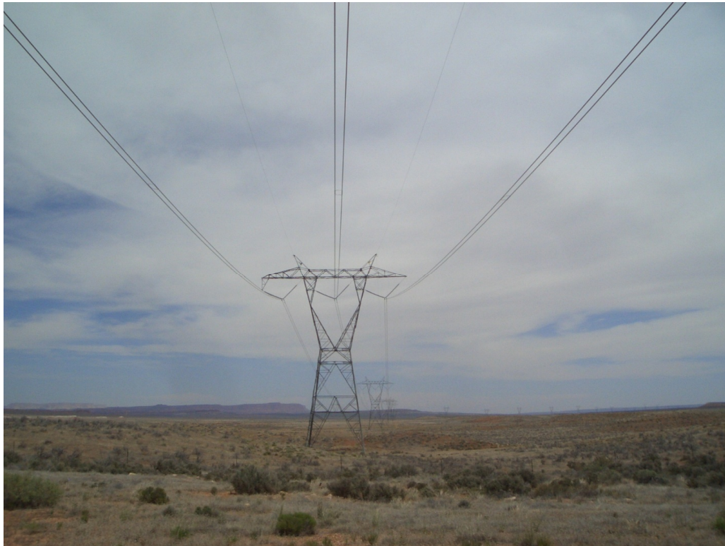
Figure 1.2 Self-supported transmission tower (Source: Wikipedia: http://operationcircuitbreaker.wordpress.com/chapter-4-transmission-line-vulnerabilities )
