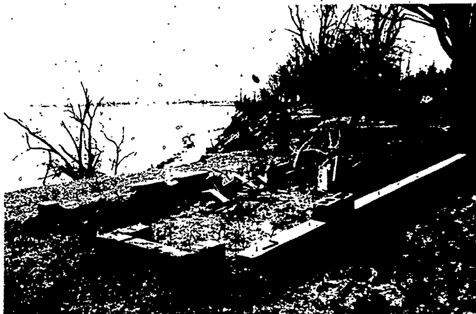
FIGURE 19 View of the Erie shoreline at Port Burwell, showing the foundation of a cottage that has been relocated. Relocation and structural set-backs are possible adjustments to shoreline erosion.
