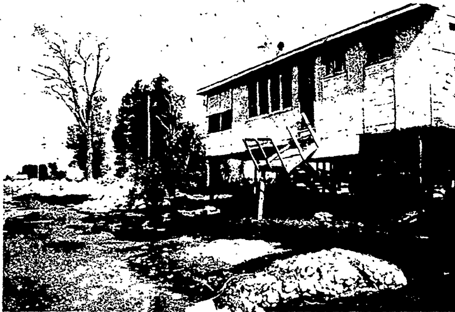
FIGURE 6 View of the Long Point sandspit, showing an area of shoreline that is undergoing serious erosion. The sand dune upon which this cottage was built has been washed away by storms.
