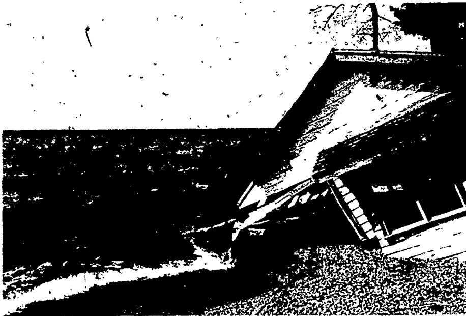
FIGURE 12 View of shoreline damage at Rondeau. About 30 cottages in the Erie Beach area were destroyed by the fall 1972 and spring 1973 storms.
