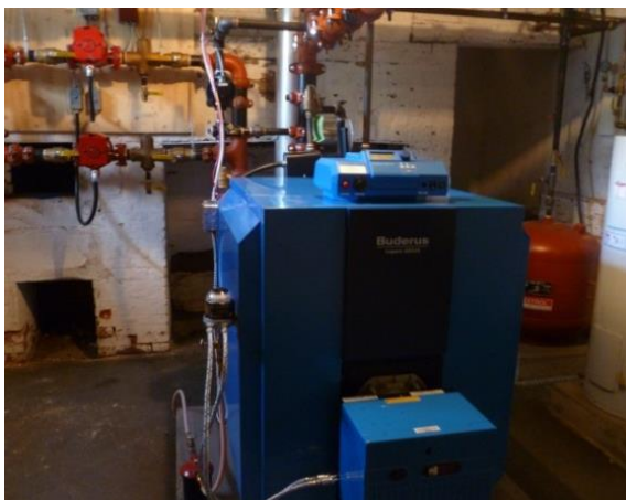
Figure 3.15: In the basement at Prescott House & Gardens Museum (Photo by the author, 6 October 2012).
