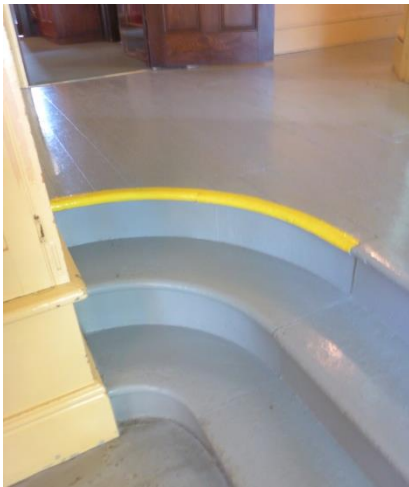
Figure 1.16: Yellow paint marking a change in elevation at Eldon House (Photo by author, 24 September 2013).
