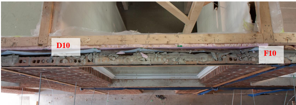
Figure 5.1 - Wall D10 - F10 before loading.
