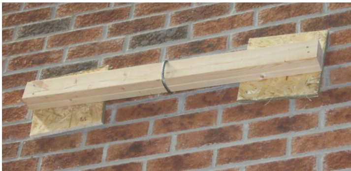
Figure 3.12 - A load pad for positive loading.
