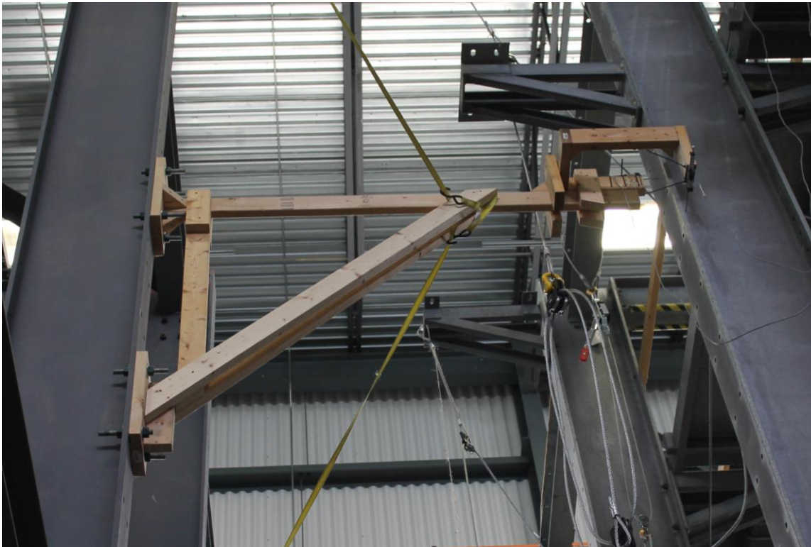
Figure D1- Built frame for recording reaction frame movements
