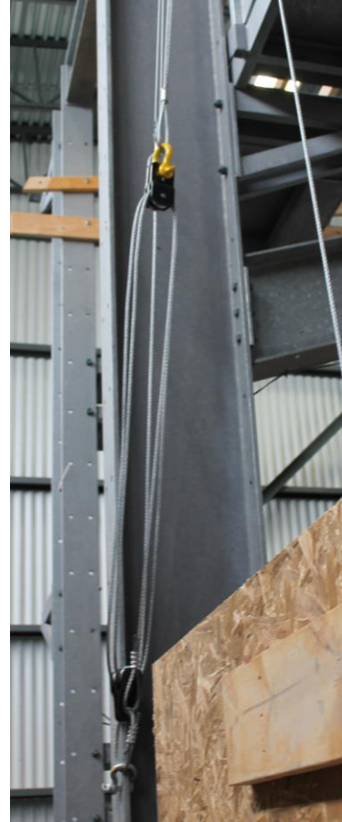
Figure 3.11 - Pulley Array in fully extended position.
