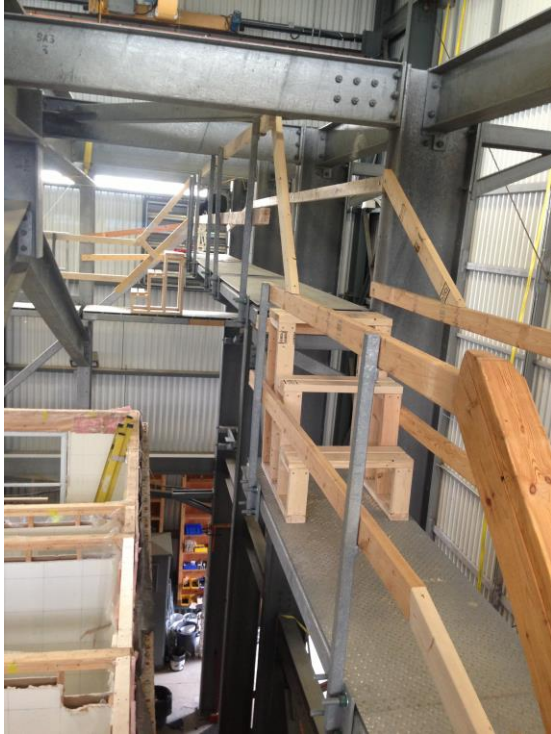
Figure 3.22 - The catwalk on the West side of the house, looking South.
