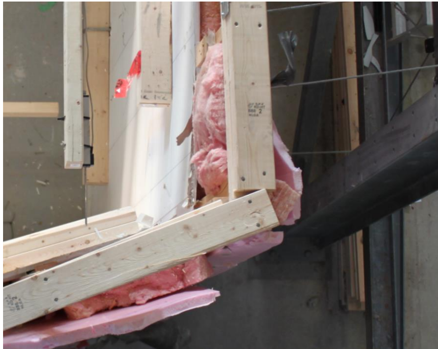
Figure 7.1b and 7.1 c – From left to right, the corner located at A1, progressively throughout the test with no brick veneer. The far right picture is after failure.
