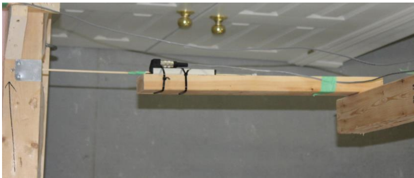
Figure I6 - LVDT W5 in place.
