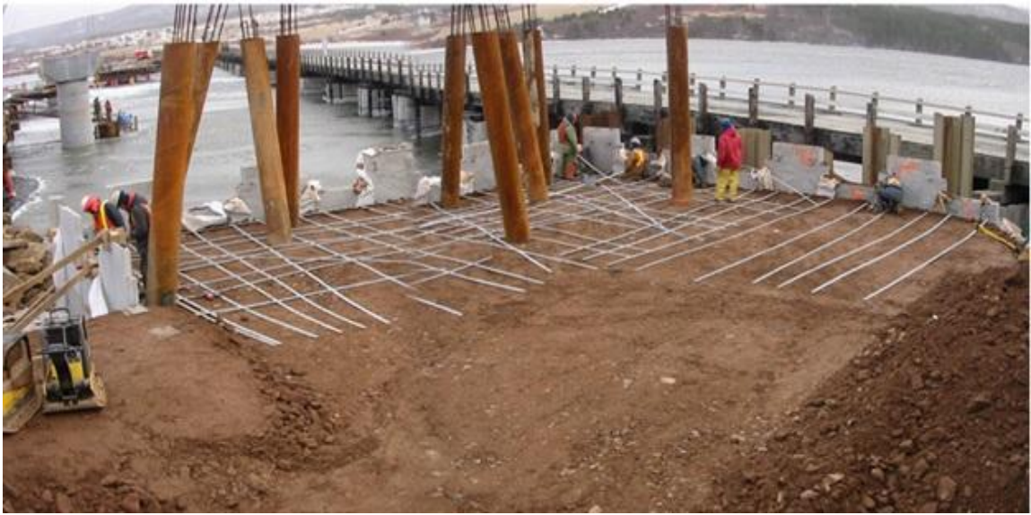
Figure 1-3 Reinforcement strips extending from a mechanically stabilized wall during construction ( www.recocanada.com ).
