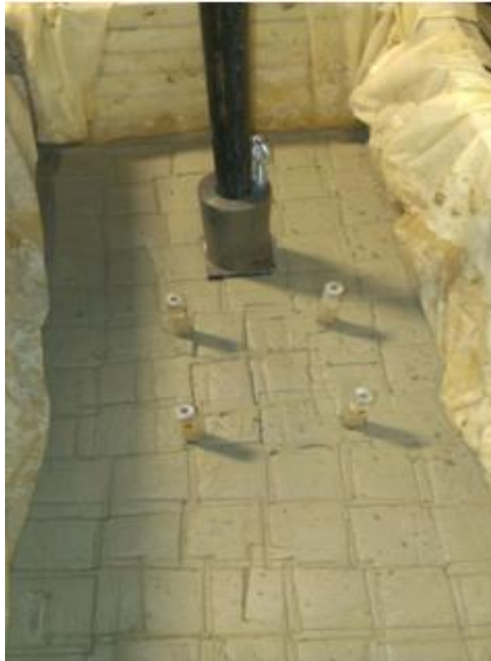
Figure 2-3: Compaction of modified glyben
