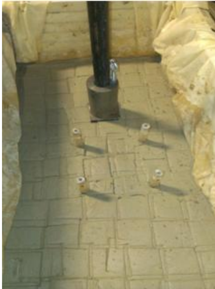
Figure 3-7: Compaction of Modified Glyben
