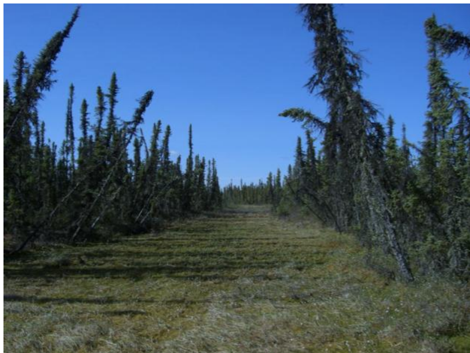
Figure 1-5. Picture showing a winter road cleared in 1943 west of Goose Lake in Scotty Creek. Surrounding trees are beginning to lean due to a loss of load bearing capacity as a result of permafrost thaw (Williams, 2013).
