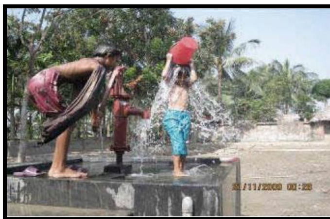
Figure 3: Tube well with raised concrete platform.
