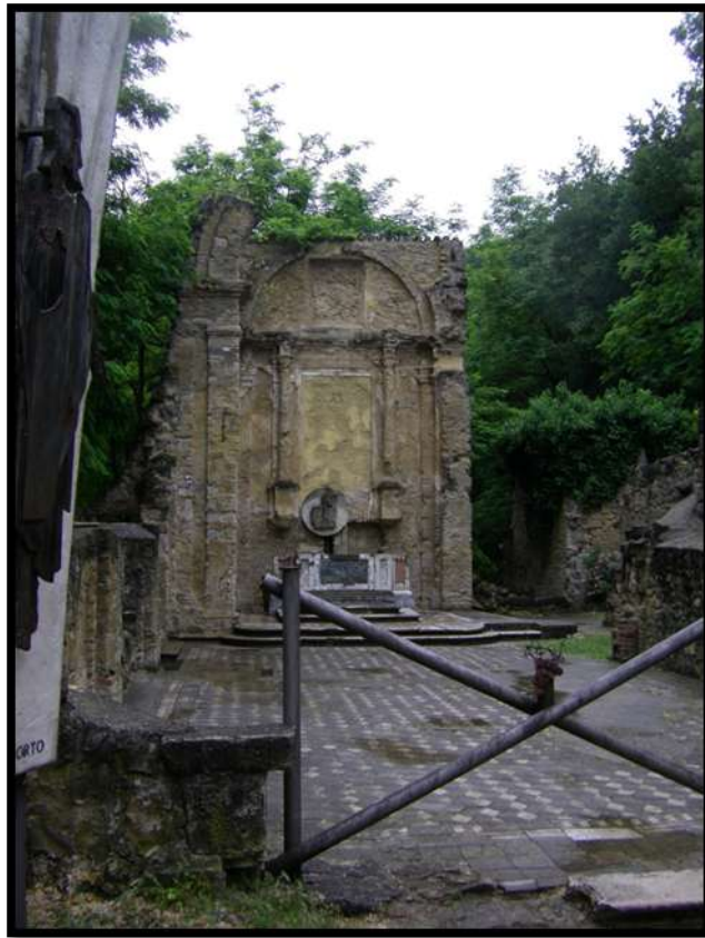
Casaglia Church is still used for services. Since this picture was taken in 2007, the walls on the back right have been reinforced to prevent them falling down. (Author photo)
