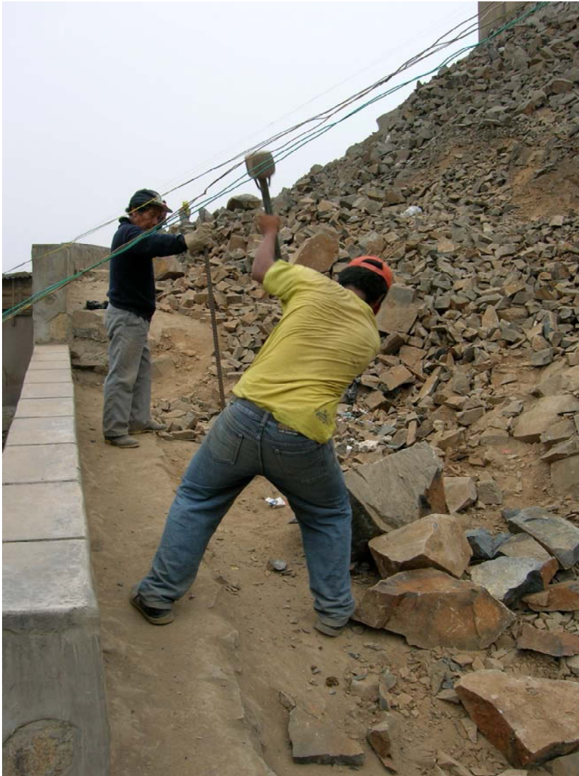
Two men breaking up rock that has been pried and sledge-hammered out of the hill. Usually, a retaining wall is built first, then rock is tumbled out from beside the wall to form the base of a road. Many of the access roads have been built in this fashion. Men often do the heavier work like that shown above. Excess rock is being broken up to be taken away in dump trucks. Photo: author
