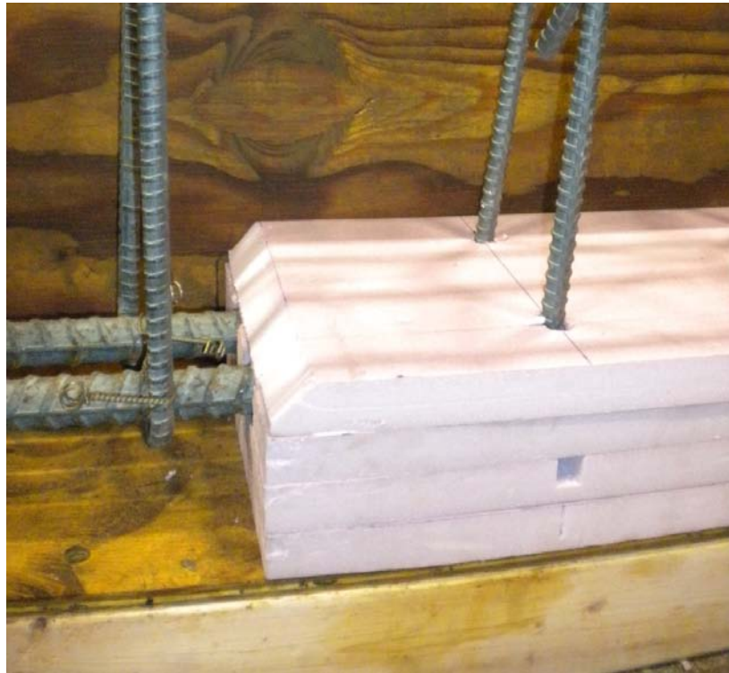
Figure 4-9: Foam Insulation Void Enclosing the Flexural Reinforcement.
