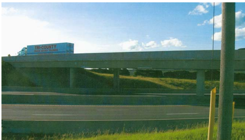
Figure C-3: Cedar Creek Road Underpass Bridge (MTO 2010).
