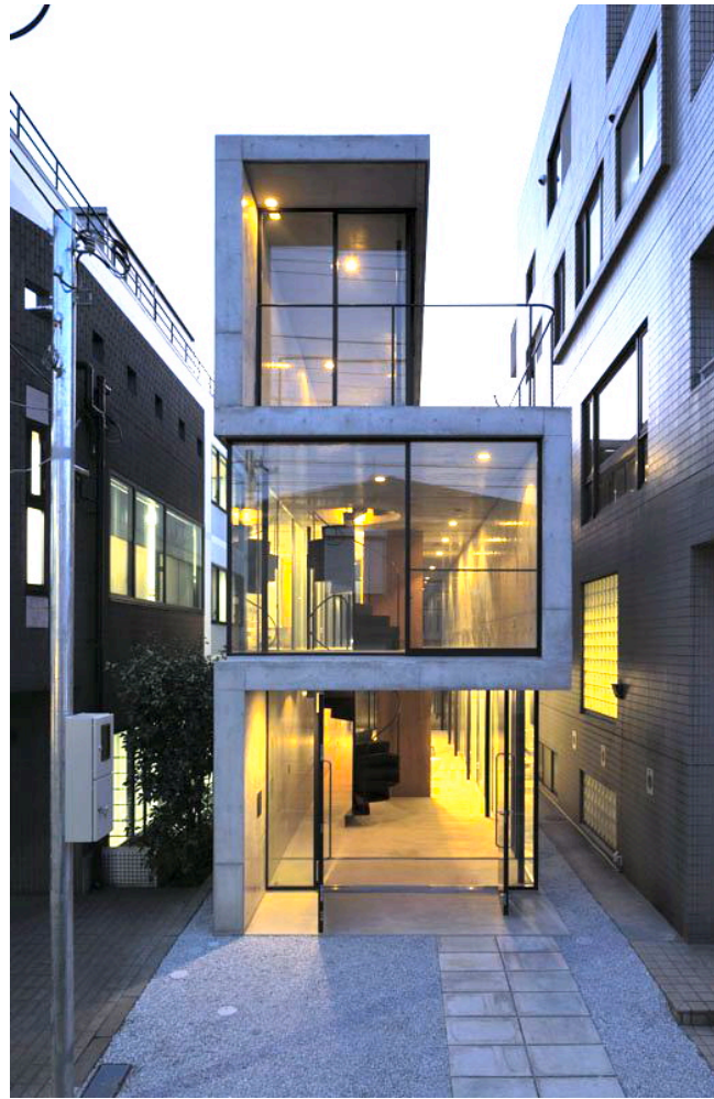
Figure 5: Florian Busche Architects’ “The House in Takadanobaba” (2011) by Hiroyasu Sakaguchi, Tokyo, Japan
