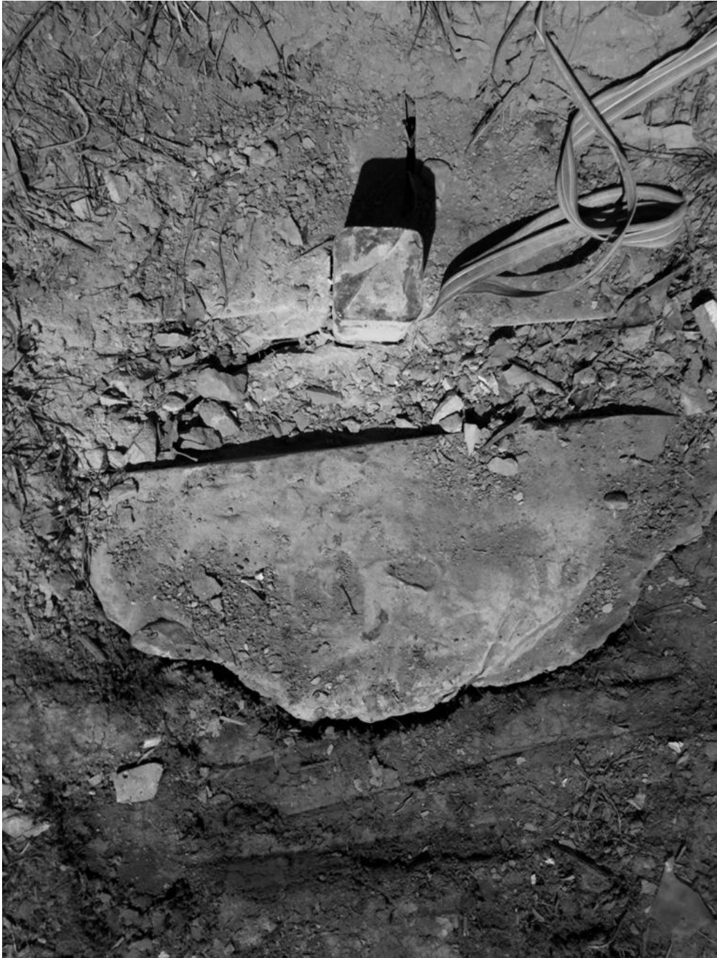
Figure 6.6: (a) Gap opening behind the pile-RHPM, static test; (b) Radial cracks profile at end of static test-RHPM.
