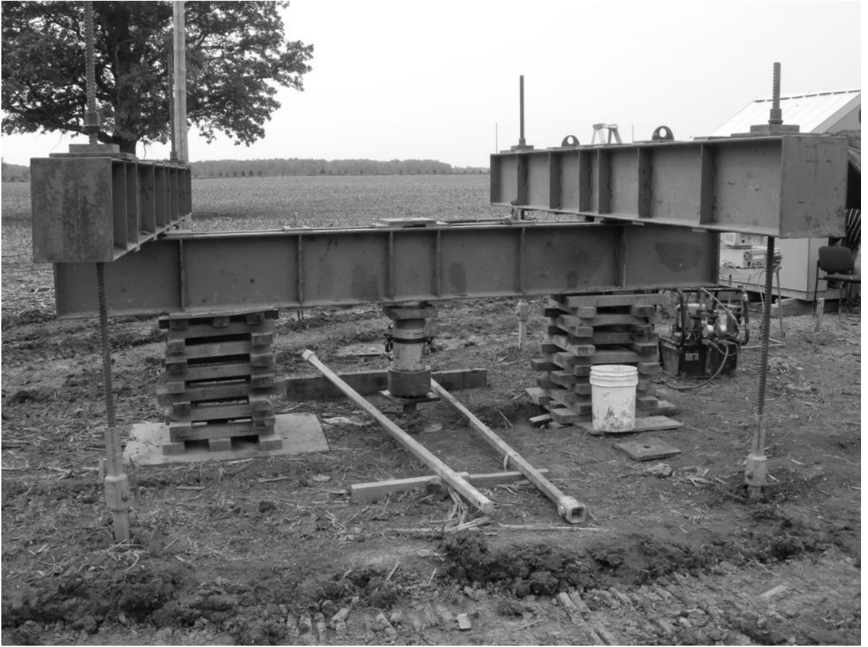
Figure 3.3. Full view of axial load test set-up.
