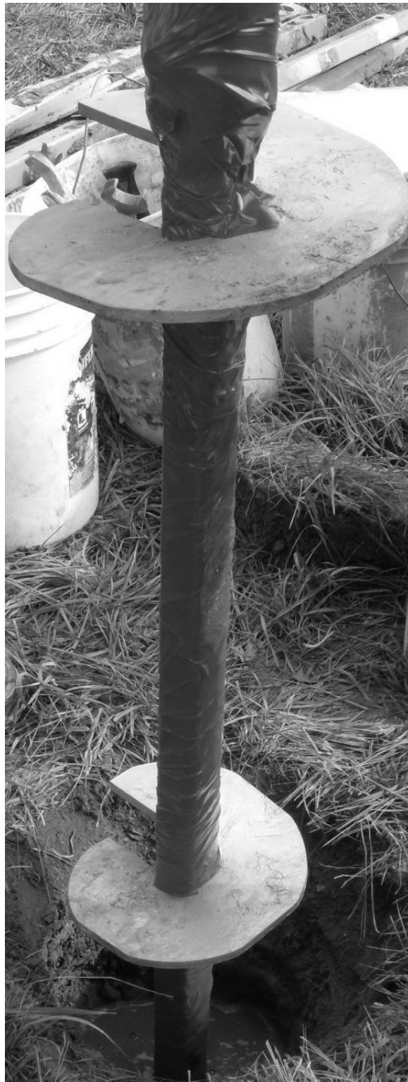
Figure 3.2. (a) Strain gauge installation. (b) Strain gauge protection through tape.
