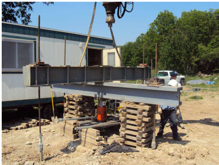
Figure 6. 5. Centering and leveling the upper beam over the lower one
