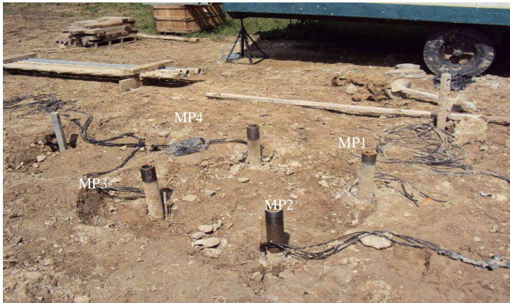
Figure 4. 14. A group of four micropiles
