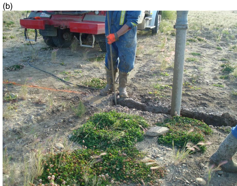
Figure 4- 3: Digging the open trench using hydro-dig technique
