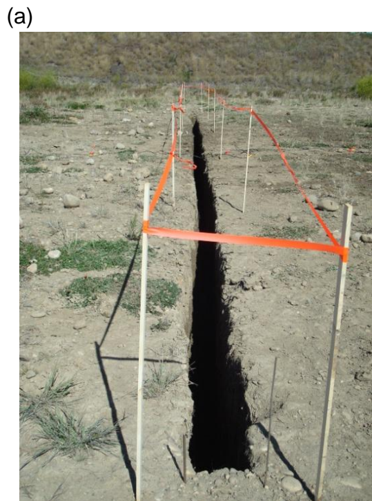
Figure 4- 8: Trench barriers after construction completion (a) open trench and (b) in-filled geofoam trench
