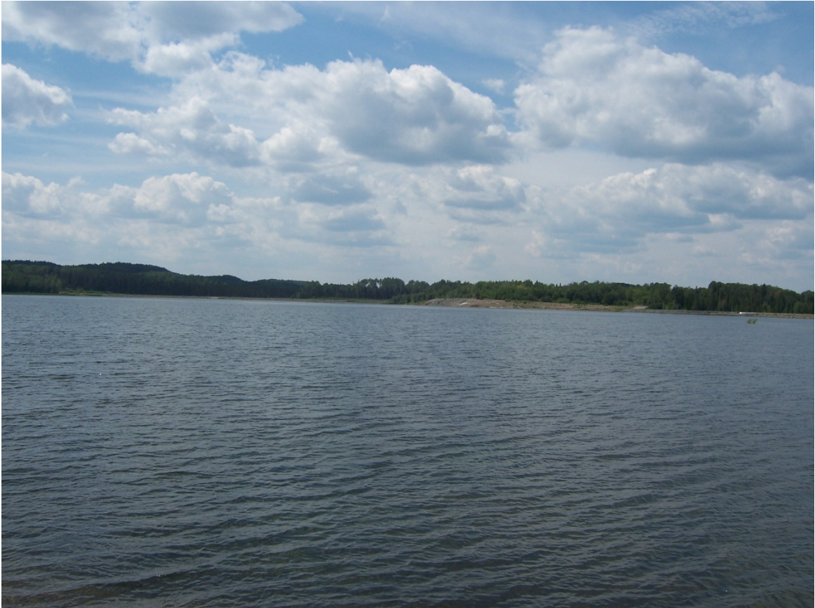
Figure IV-1 Shebandowan Mine tailings storage facility, located near Thunder Bay, ON, Canada
