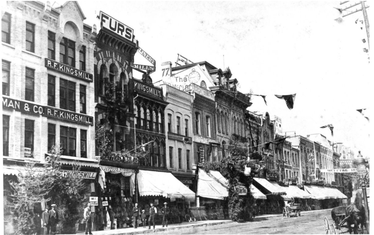
FIGURE 5.22 Traveling eastward the buildings are built at a later period and have more ostentatious designs.
