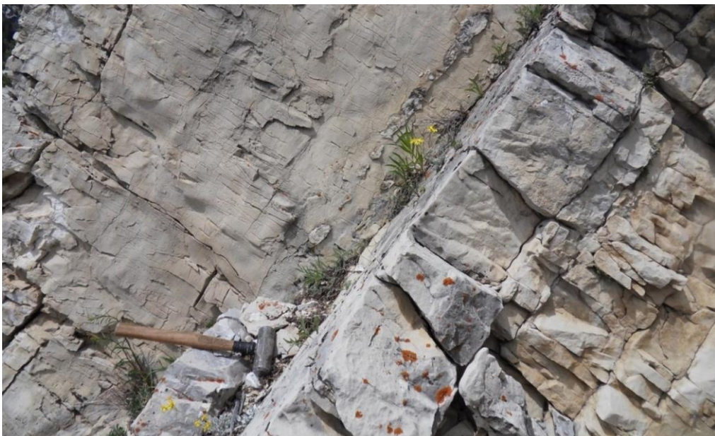
Figure 4. 19 Fracture development in Allan Member Limestone at the back of the Norwegian Thrust.
