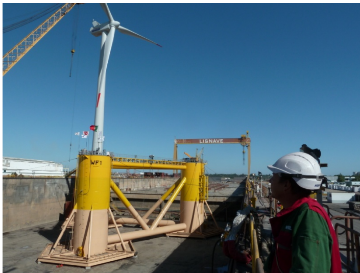
Figure 2-51: Windfloat prototype under construction in 2011 in Setubal, Portugal
