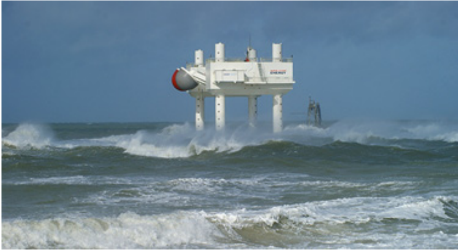
Figure 2-31: Wavestar in storm protection mode at Hanstholm
