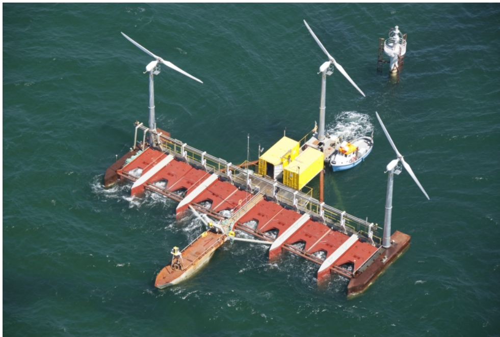
Figure 2-59: FPP Poseidon 37 1:6 scale device at sea
