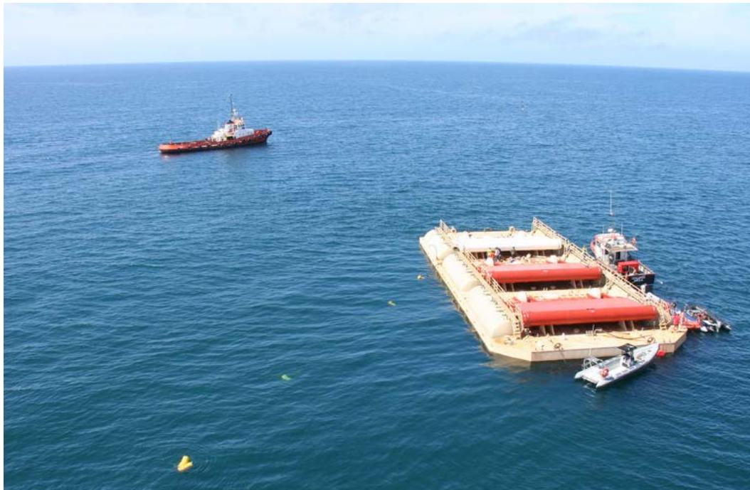
Figure 2-37: Deployment of the 300kW WaveRoller Unit
