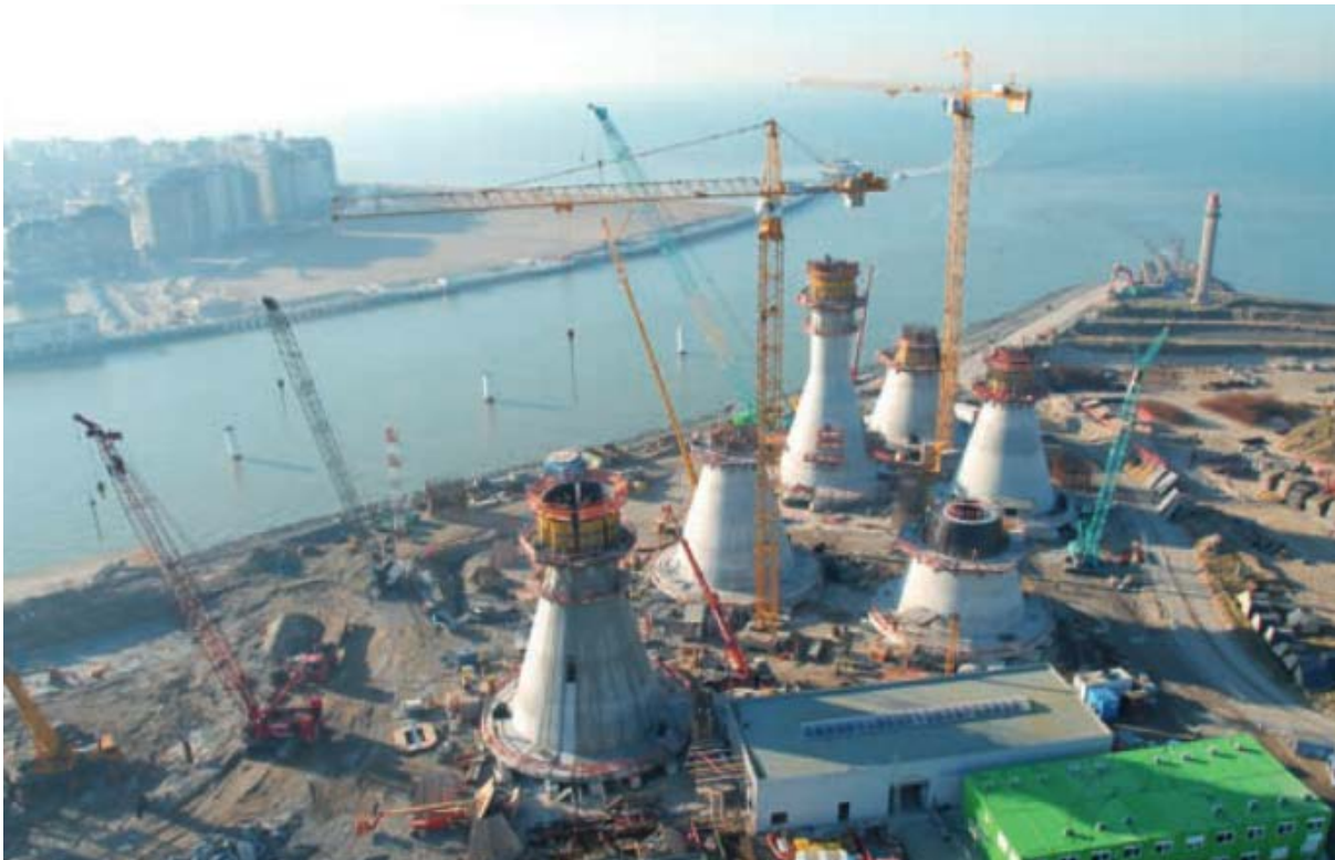
Figure 3-21: Thornton Bank GBS Foundation Port-side construction site
