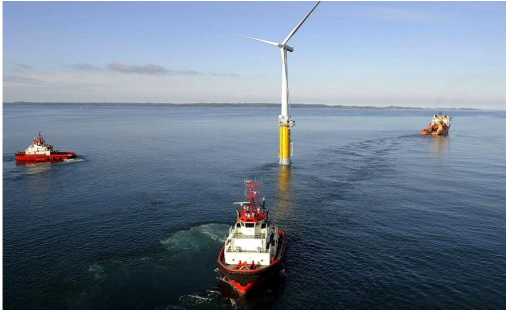
Figure 2-57: Hywind foundation following final installation at Karmoy
