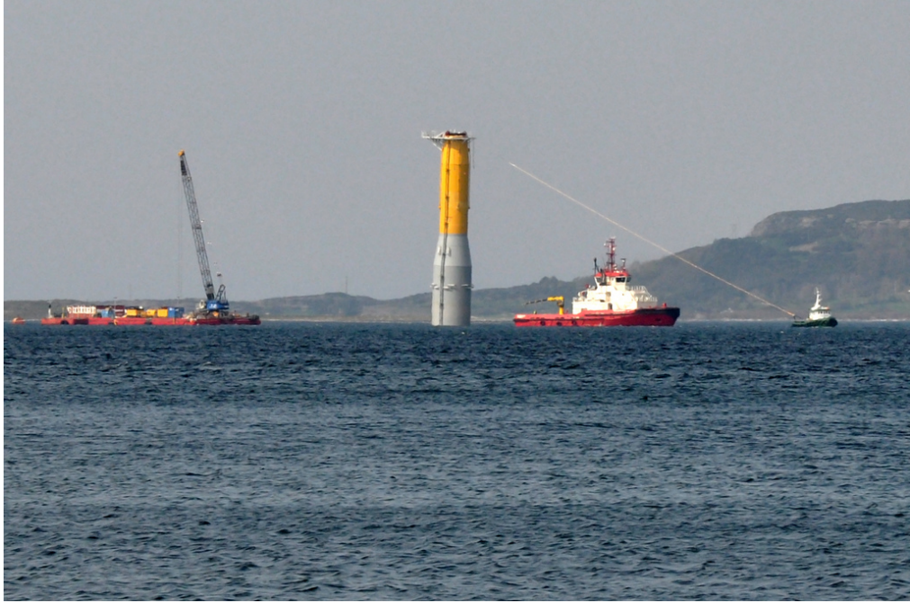
Figure 2-55: Hywind foundation during “upending” procedure
