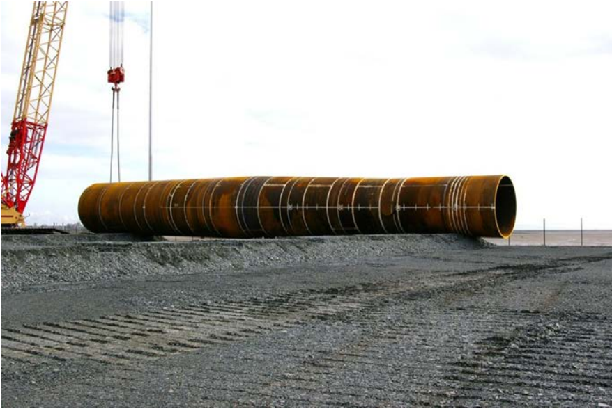
Figure 3-14: Completed Monopile
