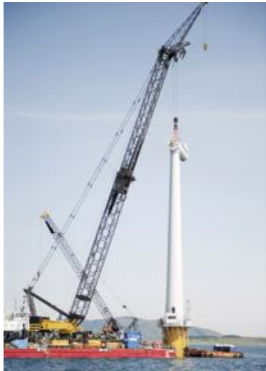
Figure 2-56: Hywind foundation during wind turbine installation
