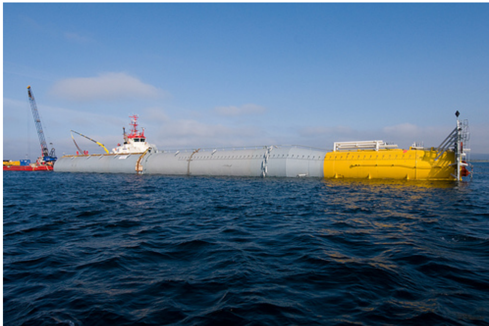
Figure 2-54: Hywind foundation during tow-out
