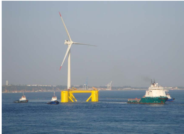
Figure 2-52: Towing of the Windfloat from Setubal by the AHT
