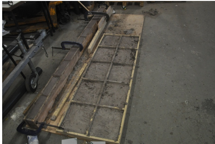
Figure D.3: Casting of concrete ballast blocks
