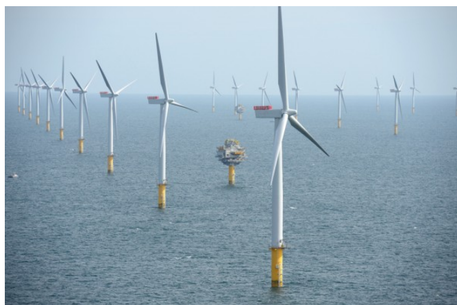
Figure 1-1: London Array monopile offshore wind farm in the Thames Estuary [3]
