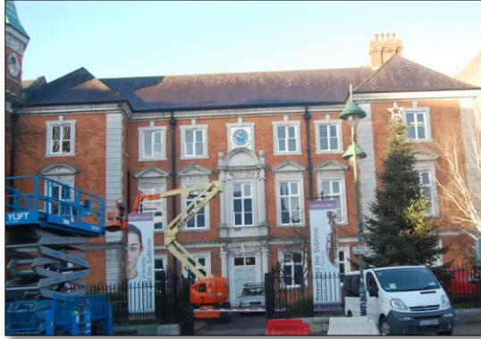
18 th Century façade of the Customs House, now Crawford Art Gallery
