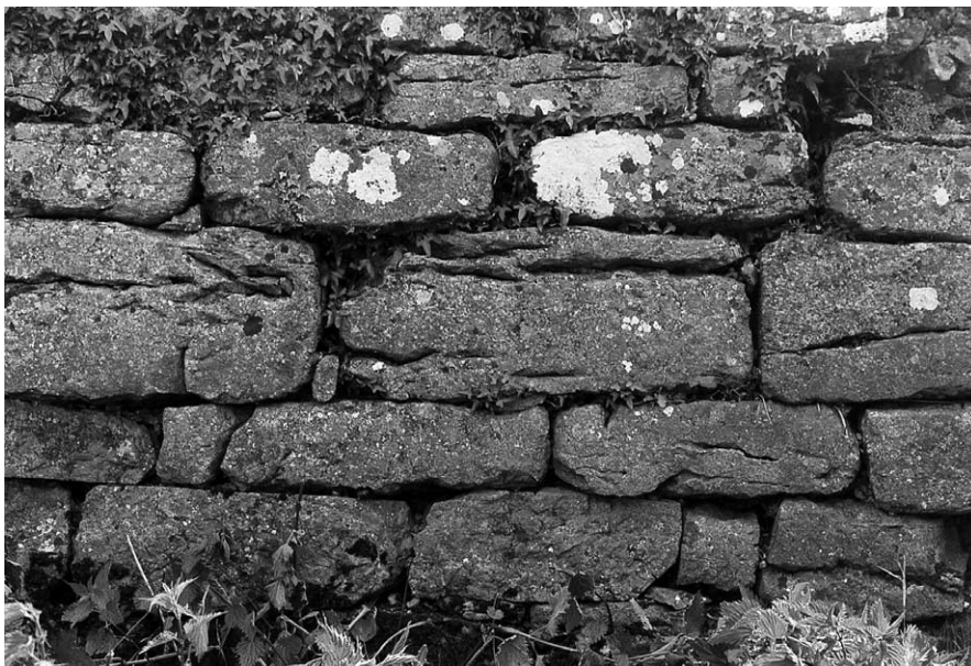
PL. VI—Masonry shot of Kilkeeran, Co. Galway. Example of the Lough Corrib/Lough Mask style.
