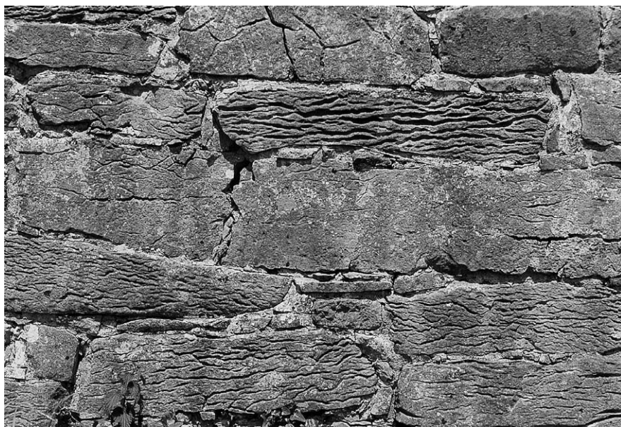
PL. V—Masonry shot of Kilcanonagh, Co. Galway. Example of the Aran Islands style.
