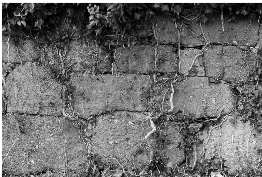
PL. IX—Masonry shot of Tybroughney, Co. Kilkenny. Example of the East Munster style.
