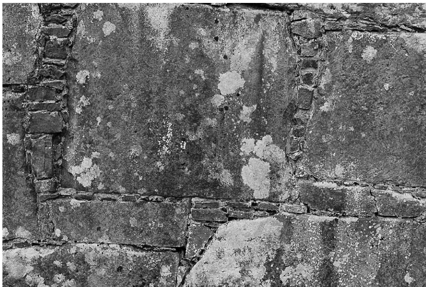
PL. IV—Masonry shot of Temple MacDuagh, Co. Galway. Example of the Aran Islands style.
