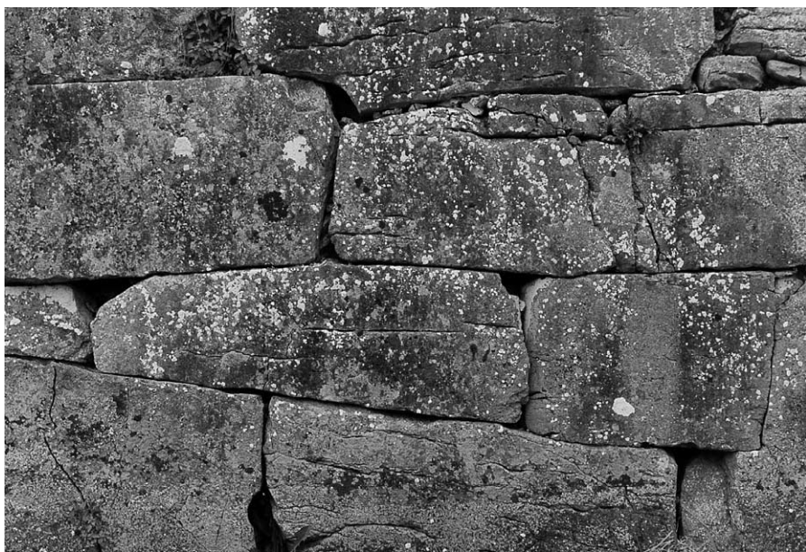
PL. III—Masonry shot of Killeelig More, Co. Galway. Example of the north Clare/southwest Galway style.
