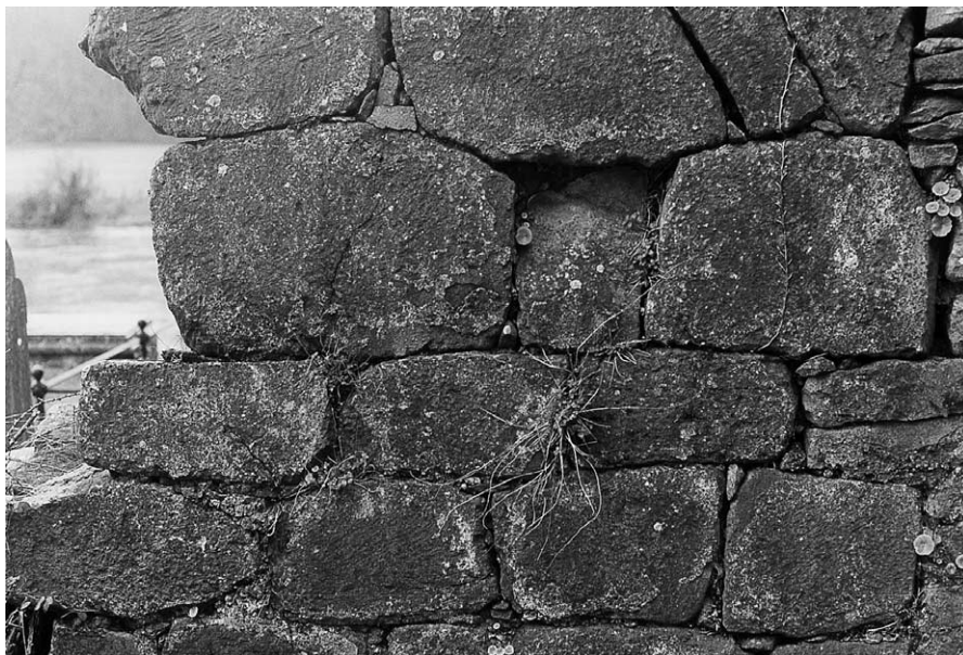
PL. VIII—Masonry shot of Kilsheelan, Co. Tipperary. Example of the East Munster style.
