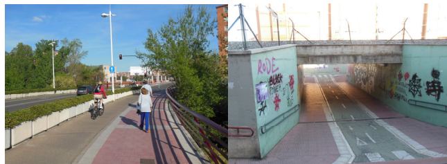
Fig 9 - Bridge on a river and below the train tracks.
