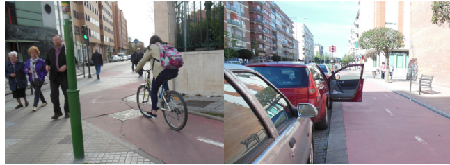
Figure 6 - Design with sharp turns, poor visibility and limited distance with designated on road parking areas.
