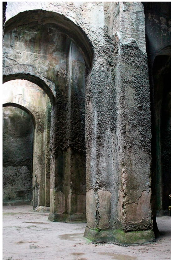
Figure 4. Status of the structure of the piscina mirabilis that should be restored to eliminate fungi and bacteria and make the place healthier for visitors.
