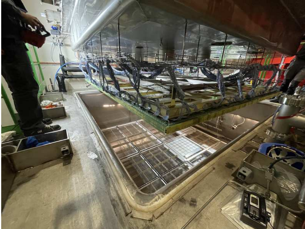
Figure 1.9. The cold box during installation of a CRP. The cathode is visible on the bottom, with an X-ARAPUCA PD installed.
