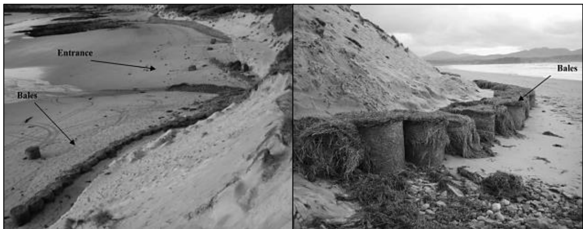
Figure 3.3: Straw bales used as a form of coastal protection. Font: O'Connor et al. , 2010.
