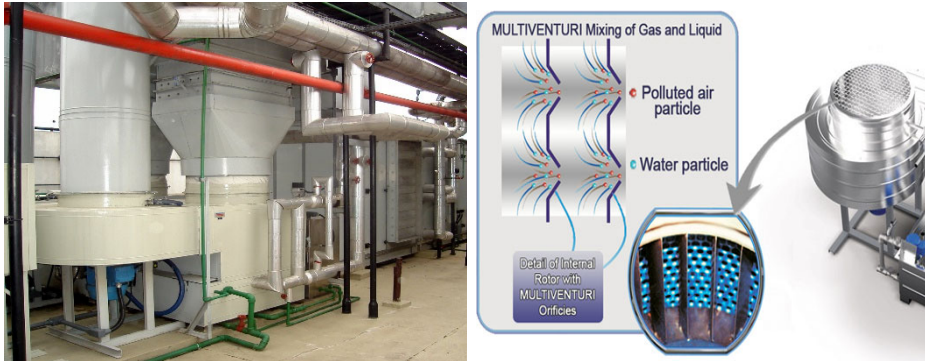
Figure 4. Hydrodynamic precipitator and multi-venturi internal detail of the simultaneous centrifugation of liquid and air in a limit load rotor. Source: Flavors laboratory, São Paulo, SP/Brazil.
