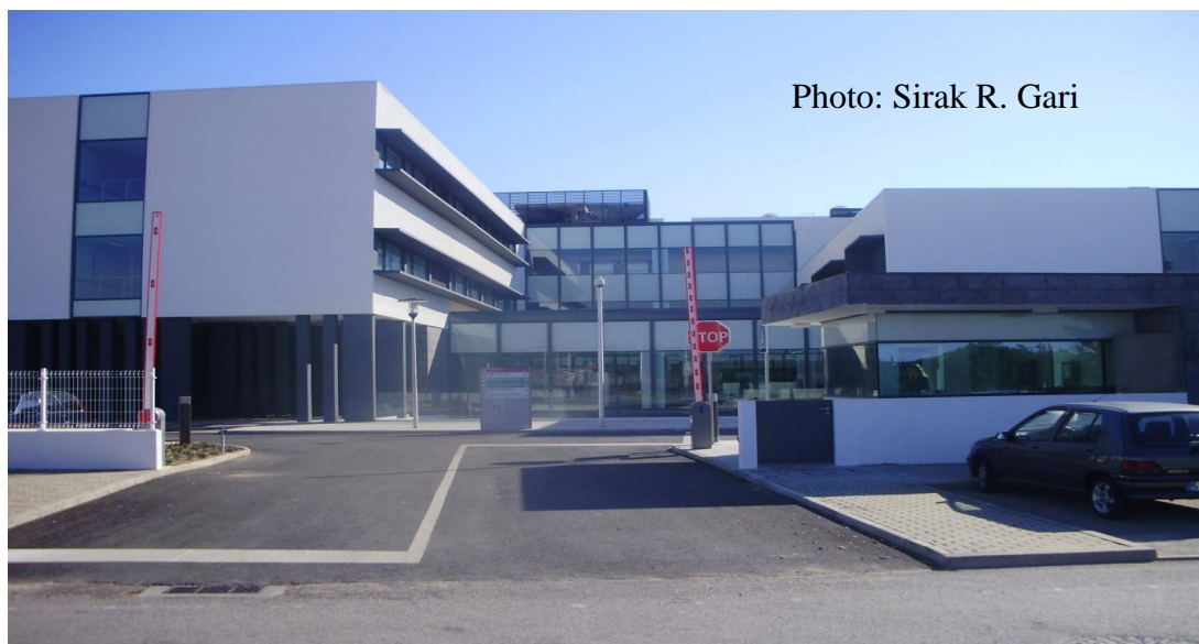
Figure 4-15: Hospital Particular Do Algarve.
