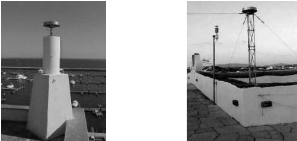
Figure 2.7 Cascais (left) and Lagos (right) stations panoramic views.
