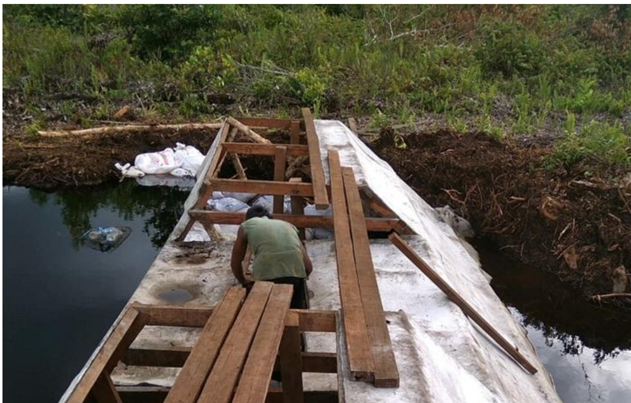
Figure 2. Installation of a canal block in Tumbang Nusa.
