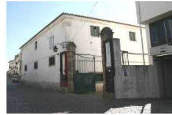
Figura 372 – Fachada Norte e portão principal [LEB (2010c)]
