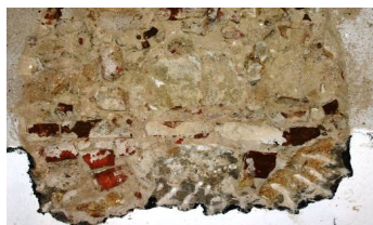
Figura 380 – Parede de alvenaria interior [LEB (2008)]
