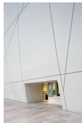
Figura 99: Darwin Center, C.F. Møller Architects. Fonte: http://www.archdaily.com
