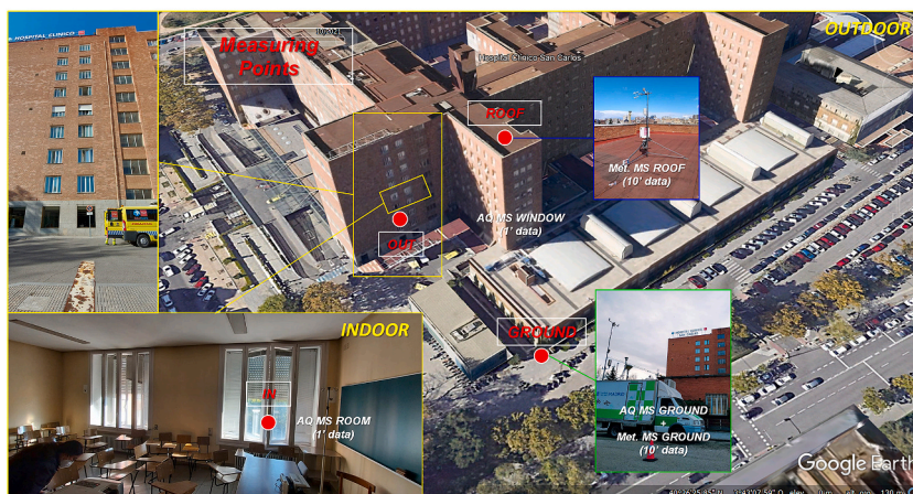
Fig. 1. Right) San Carlos Hospital (Madrid): outdoor view. Left up) Location of some ambulances. Left down) room: indoor view. Measurements location (red points). (Source: Google Earth satellite image).
