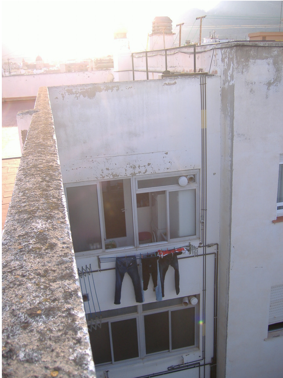
Fachada F4-PLE. Acabado exterior [Ref. FA019]
