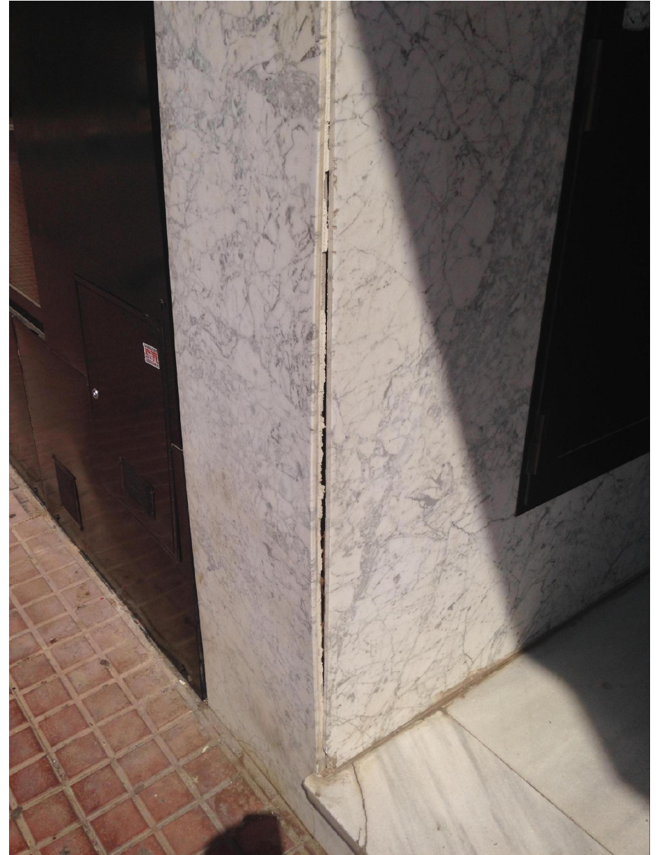
Fachada F1b. Acabado exterior [Ref. FA006]
