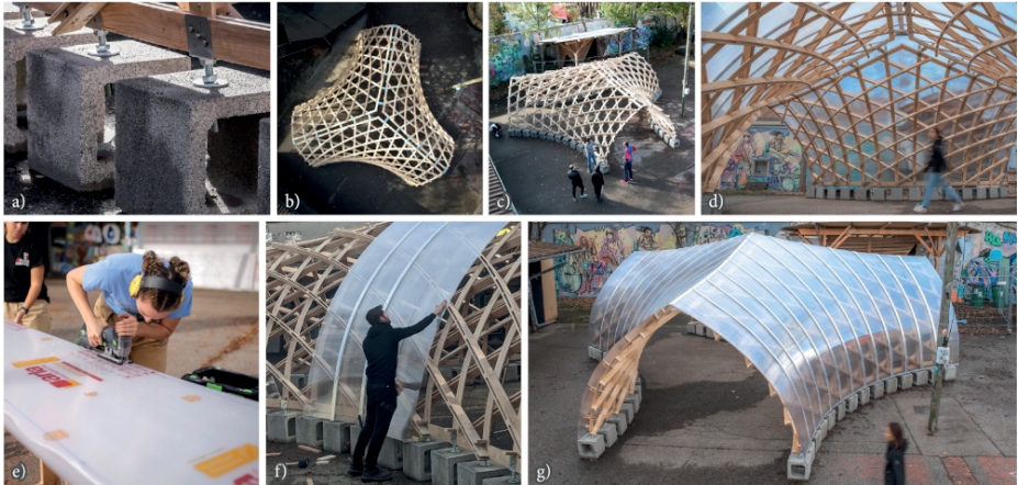
Fig. 8: Completed timber gridshell. Top Row: a) Precast concrete blocks with steel supports. b,c) Birds-eye view of the timber gridshell without cover. d) Inside the Timber Vault. Bottom Row: Polycarbonate panels are tailored with concave edge (e), and installed using aluminum mullions along the geodesic directions (f), to create a smooth, transparent skin (g).
